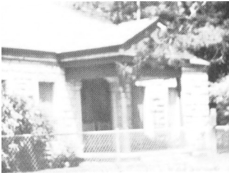
"Stonewall", 1985 Residence of Bill Gibson
